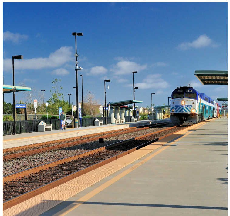
Poinsettia Train Station platform in Carlsbad
