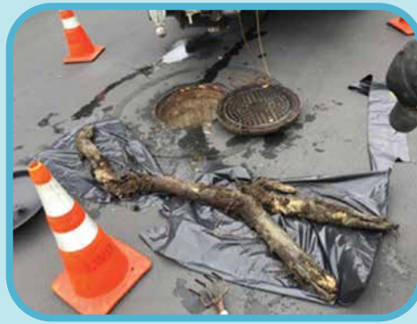
This root was discovered during our routine pipeline inspection.
