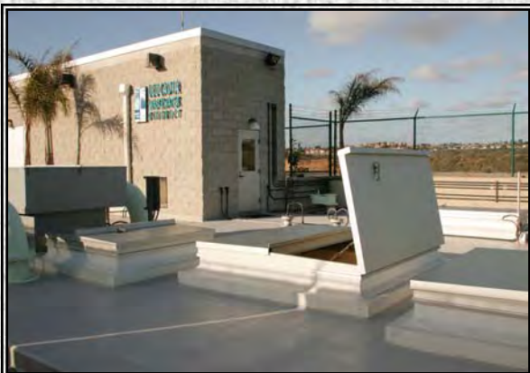
Batiquitos Pump Station
