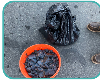
Pool plaster removed from the sewer.
