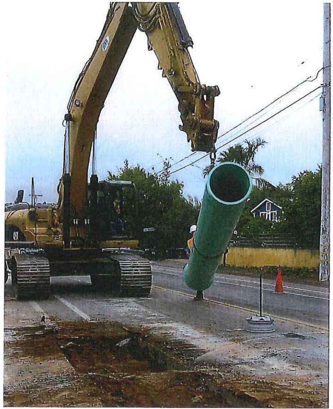
The Force Main Project Team lays down a 24" diameter PVC pipe along La Costa Avenue. Made of chemically stable polyvinyl chloride, the new pipeline will last 50+ years.
