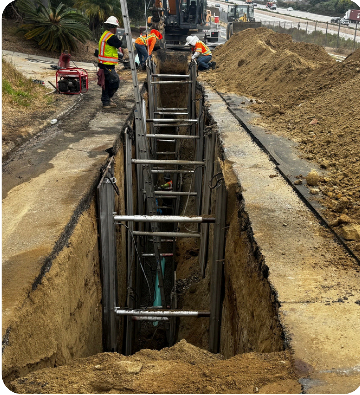
Photo: Gravity Pipeline Project
