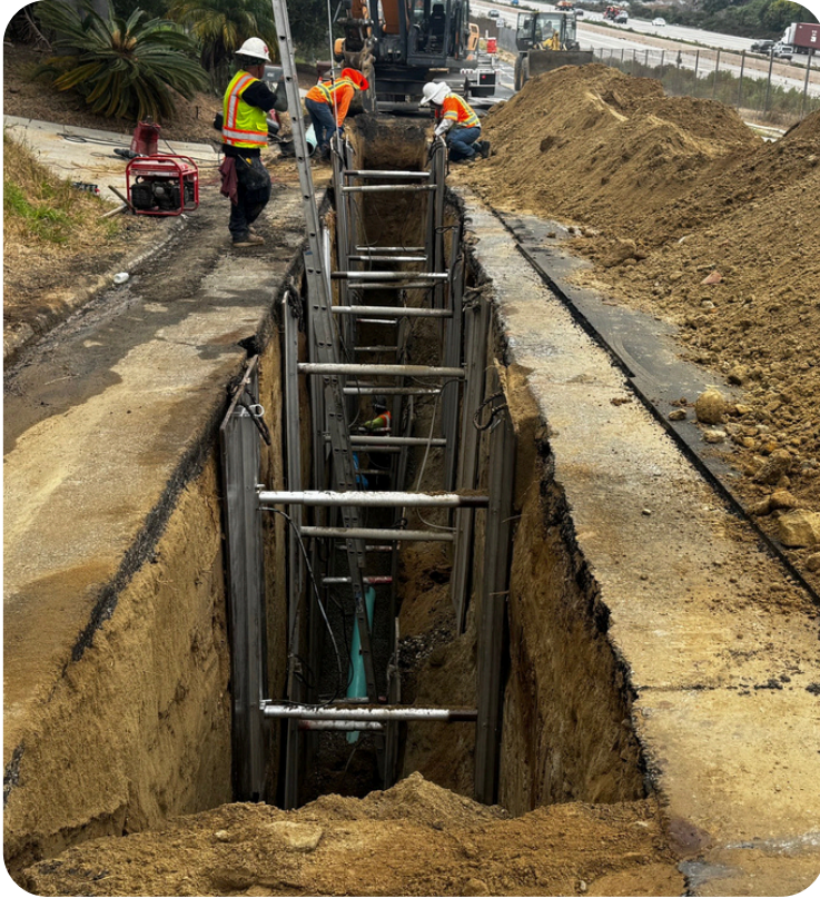
Photo: Gravity Pipeline Project
