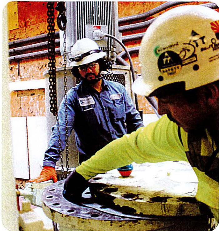
Field Services Technicians open a check value to allow the Smartball into the sewer system.
