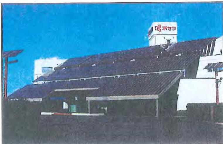
Kyocera installed a 1 kW test system at its research facility in Sakura, Japan, as early as 1984. The PV modules are still performing very well to this day and are a great source of data for R&D efforts.
