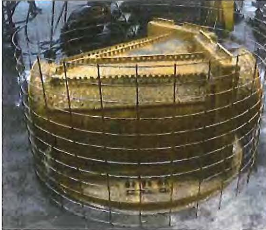
Manhole being formed around Predl liner.
