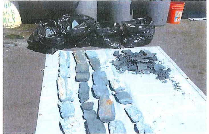
Hardened pool plaster removed from LWD sewer pipes.
