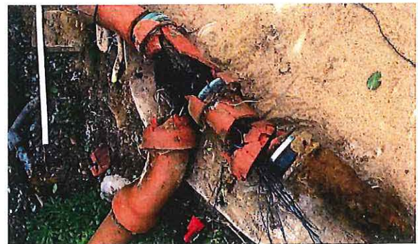
Large root inside Mr. Hooker's sewer lateral
