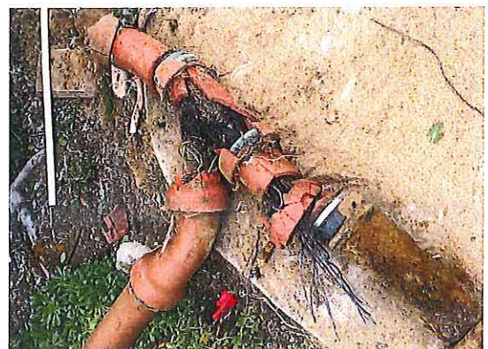
Large root inside Mr. Hooker's sewer lateral.
