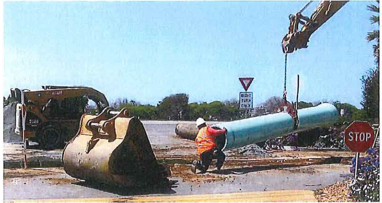
Portions of the iron Force Main was replaced with a PVC pipe due to internal corrosion
