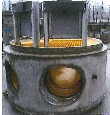
Finished precast manhole with FRP grating and gates.
