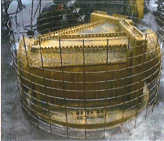
Manhole being formed around Predl liner.
